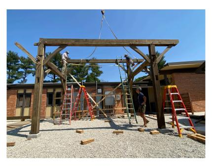
Mission Green installed a permeable paver courtyard above the French drain and below the post and beam solar pergola to better reflect on the bi-facial solar panels. A stylized cross, copied from the 1958 architectural drawing for the original building, was added to the courtyard's center. Mission Green installed architectural LED lighting and an outdoor sound system. This area will become a significant new space for events at Good Shepherd while adding to the efficiency of solar production.
