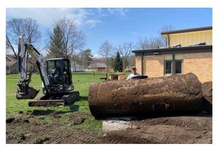
This project included excavation to a prescribed 42" depth. Unfortunately, we couldn't anticipate the size of the old fuel oil barrel in that location. It was buried nearly 7' deep and roughly 15' long, requiring filling and compacting gravel every 5" of rise. There is approximately 200 ton of compacted, crushed stone below this courtyard.
